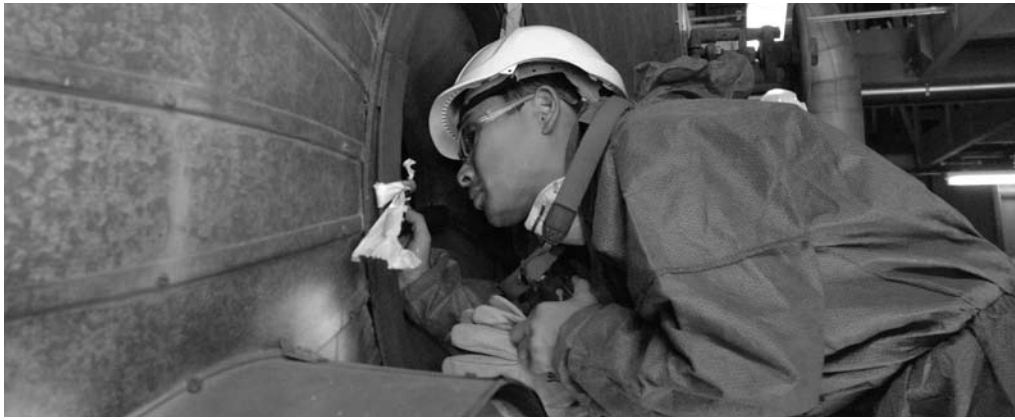
Image (left) Terutoshi Uchida from Callide Oxyfuel Project partner IHI Corporation inspects the unit 4 boiler drum during a condition assessment of Callide A in November 2006.
